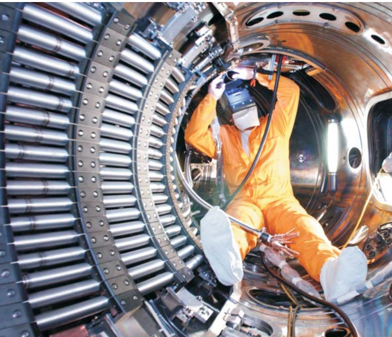
Installation work in the combustion chamber of the TEXTOR experiment
